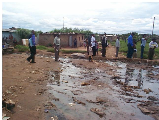
**Fig. 2.** Low earth barriers built across paths to divert floodwaters in an informal settlement in Lusaka, Zambia.
