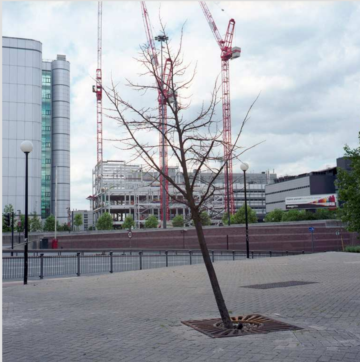
Too much concrete
